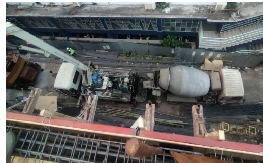
Gambar 19. Concrete Pump
