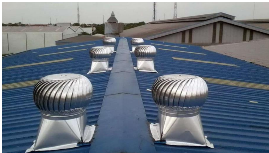
Gambar 1. Exhaust Fan Gudang Bahan Baku [4]
