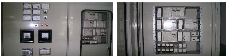
Gambar 4. Panel kontrol transformator dan Relay 42/50 MVA,150/20 kV area Tuban III
