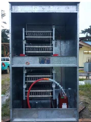
Gambar 3.4. *Neutral Grounding Resistor* PT. Semen Gresik area Tuban III
