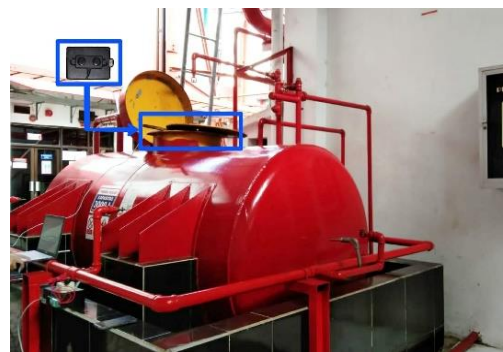
Figure 8. Sensor implementation on tank
