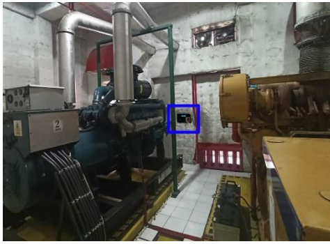
Figure 9. Implementation of hardware box in generator room
