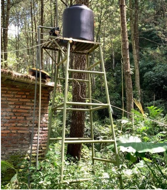
Figure 4. Placement of the water reservoir and water pump used in the toilet water distribution system at Bedengan Tourism Park Malang.
