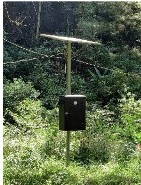
Figure 3. Installation of the solar panel pole used as the main power source for the toilet water management system at Bedengan Tourism Park Malang.
