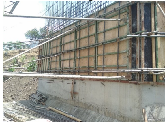
Gambar 2 Bekisting Knock Down
