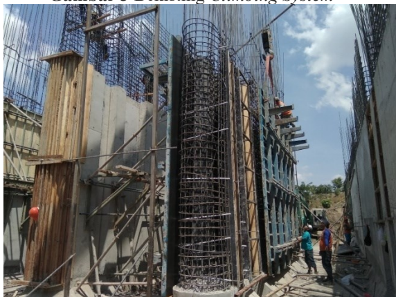
Gambar 3 Bekisting Climbing System
