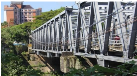
Figure 1. Side View of Steel Truss Bridge
