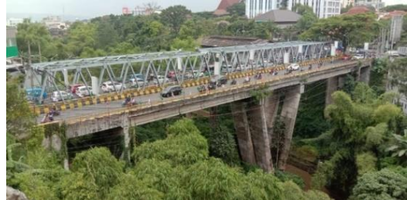
Figure 3. Side View of Concrete Girder Bridge
