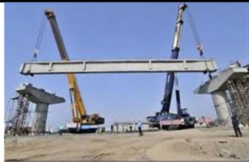
Gambar 2. Metode Girder Crawler Crane
