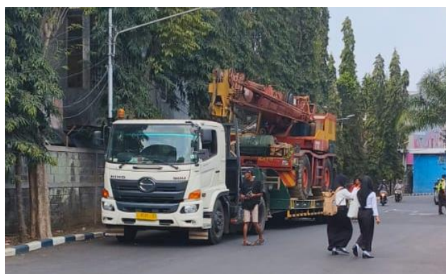
Gambar 5. Pendatangan Mobile Crane
