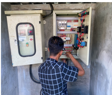
Gambar 3 Proses Perakitan Panel Kontrol Analog
