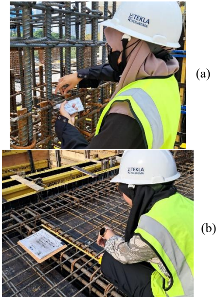
Picture 5. (a) column detail tagging; (b) beam reinforcement checking
