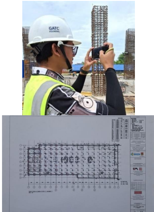
Picture 4. Weekly structural work mapping
