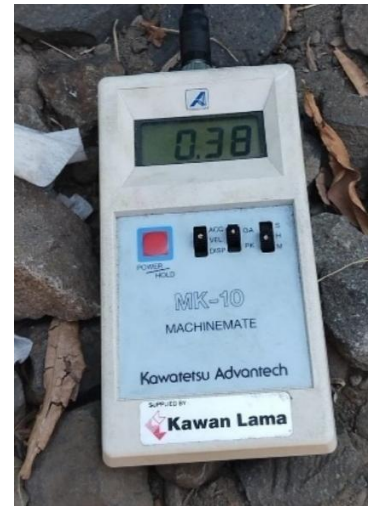
Figure 13. Testing with Vibration Meter
