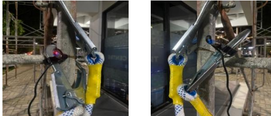
Figure 7. Safe and Unsafe Hook Positions
